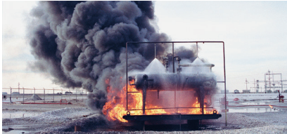
N6 nozzles protect a propane storage tank from fire and explosion.
